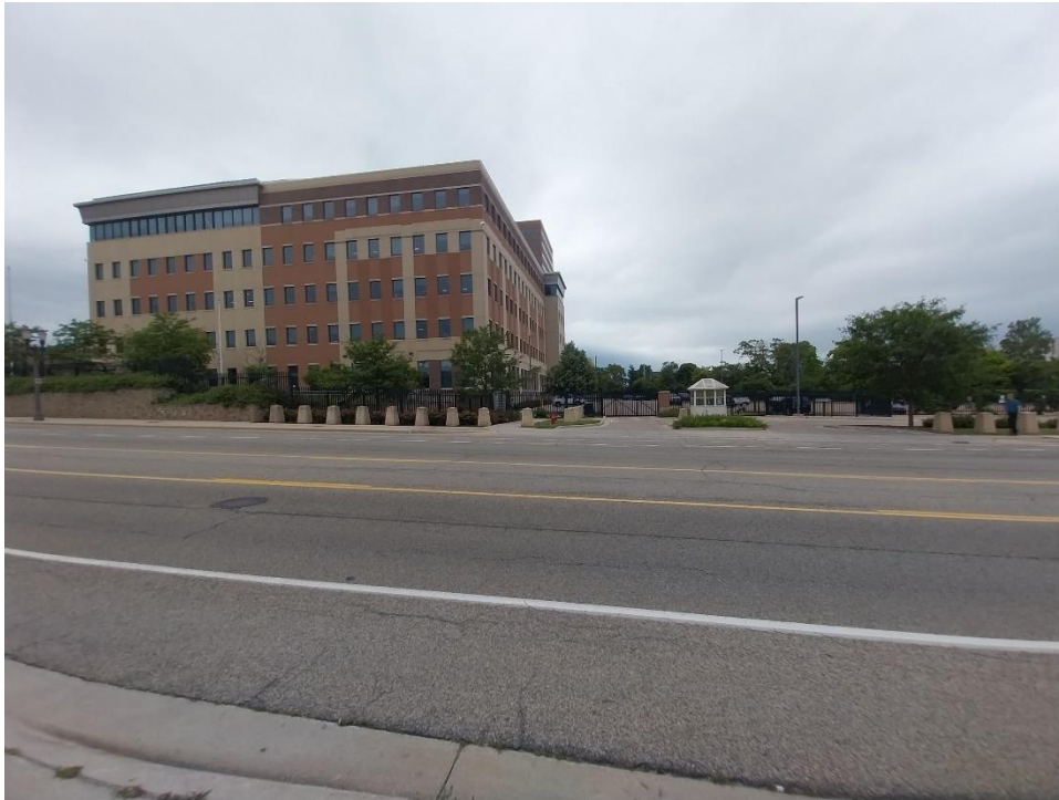
View to the North
